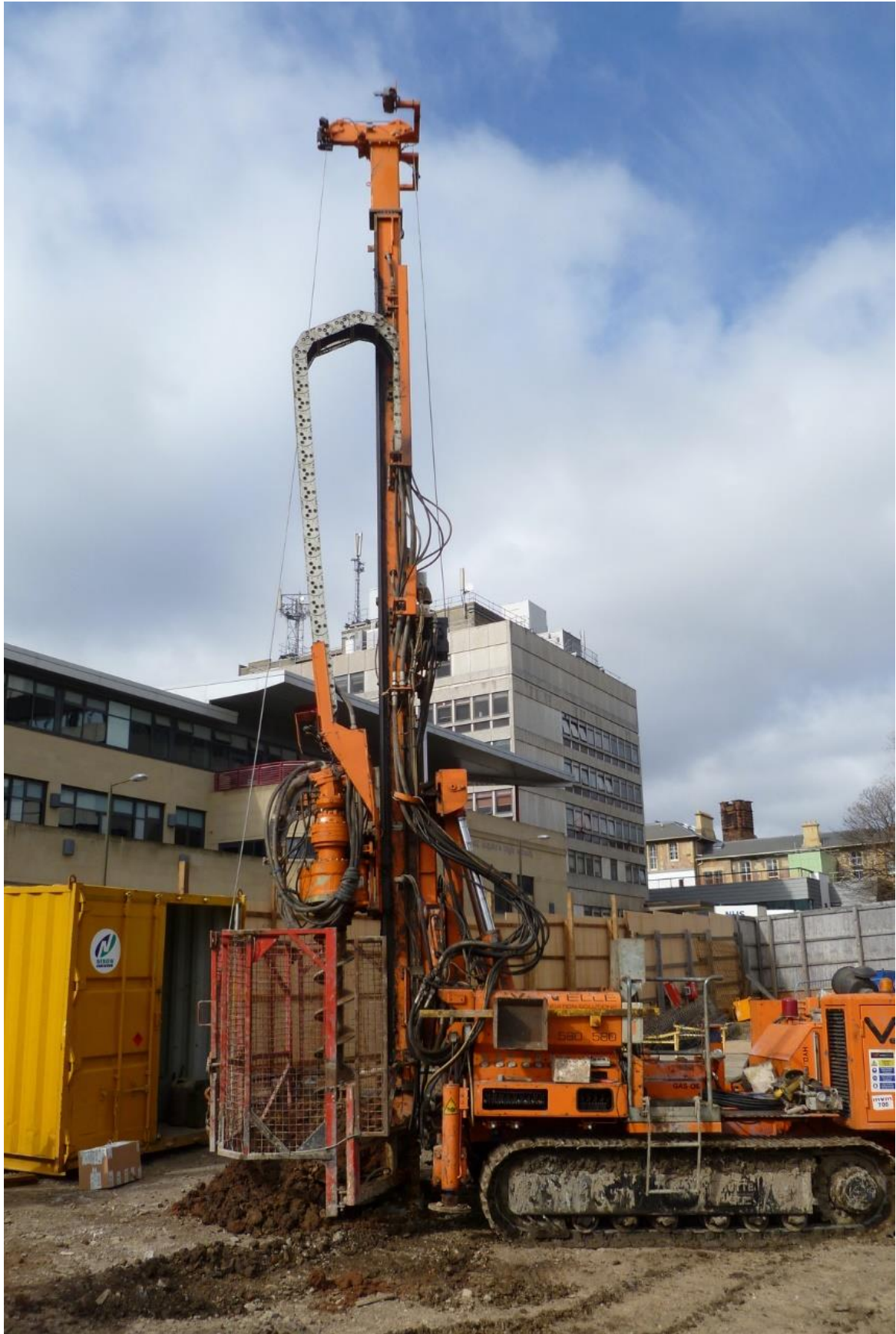
Figure 30: Photograph of an example of a piling rig
